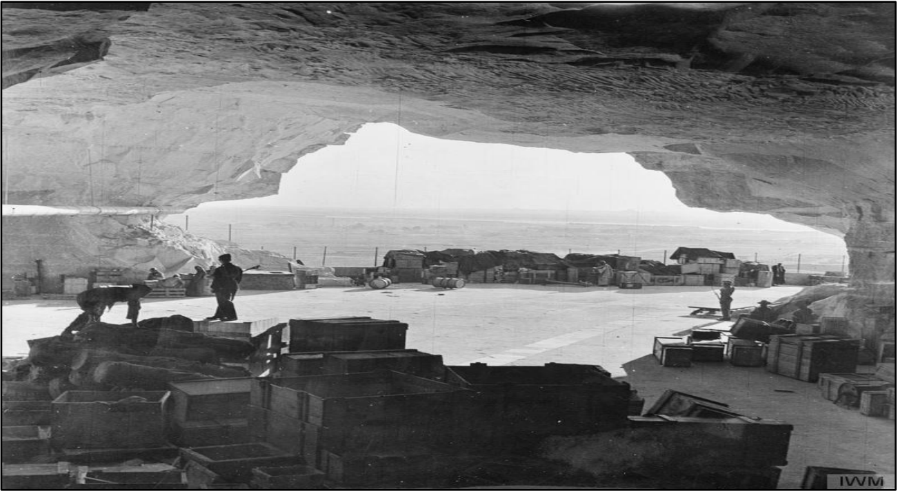
The entrance of one of the caves used as storage and maintenance workshops by No. 111 Maintenance Unit RAF at Tura-el-Asmant, Egypt. By October 1942, the RAF had established aircraft and engine repair, signals repair and general engineering sections within the caves, which also housed Army elements including 512 Army Field Survey Company RE, and a small hospital. (IWM CM 5892)
